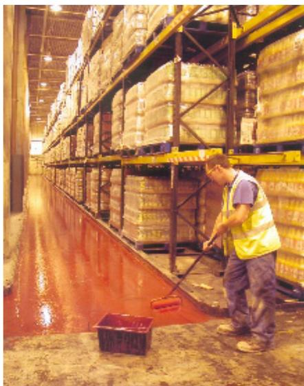
After the de-bonded screed material had been removed from each aisle, Concrete Grinding upgraded the full width of each aisle, using their unique **LASER GRINDER** process.
